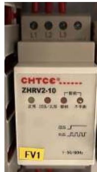
Power supply monitor
